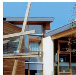
Kindergarten, Lana SANCO Solar
