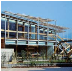
Kindergarten, Lana SANCO Solar
